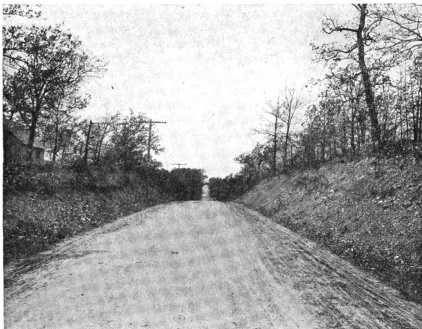
COUNTRY ROAD NORTH OF JOPLIN. BUILT BY THE JOPLIN SPECIAL ROAD DISTRICT
